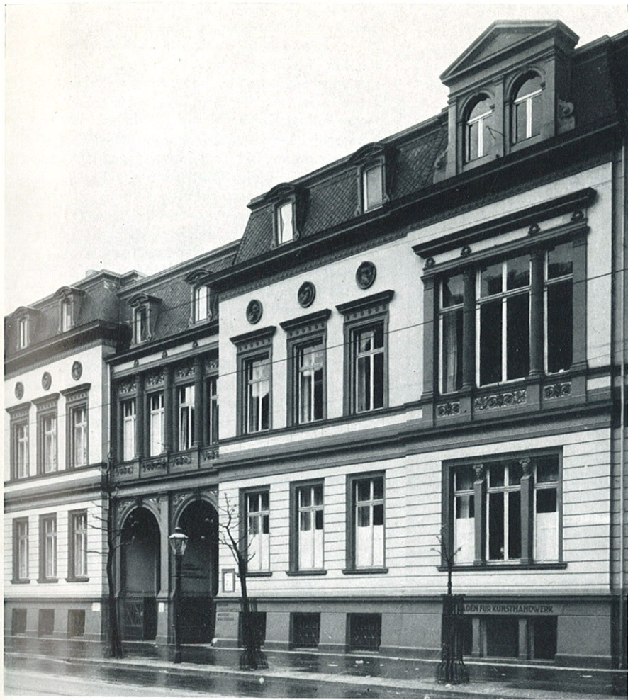
Kestner Gesellschaft, Hanover, top right-hand window, V-G's studio (1924-30) formerly the studio of El Lissitzky
